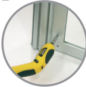
Assemble vertical profiles to the curved profile ensuring that the graphic fixing strip is adjacent to the post and facing forward (convex side).
