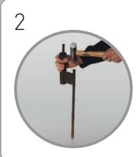
Position base where Bowhead is to be displayed. If using the ground spike, locate end of spike above desired location. Ensure strike point is directly above end of spike and, using a suitable mallet, carefully and vertically hammer into ground.
